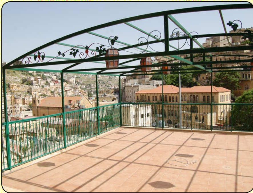
The roof terrace of the new restaurant.
