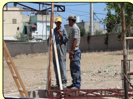
Maher(I.) is working on the sun roof.
